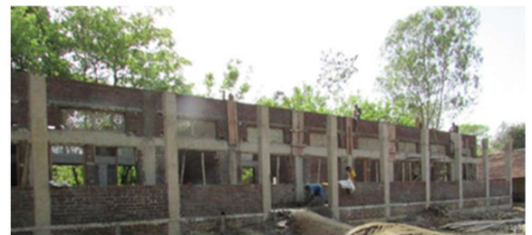
Rebuilding part of a school section that was burnt, Talasari
